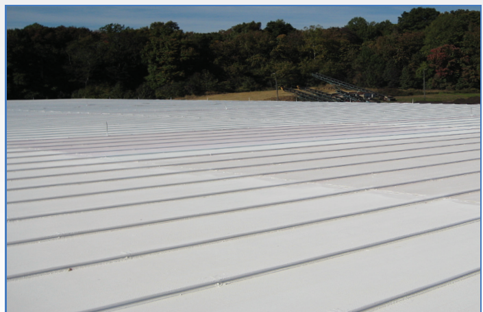
Apply 2 coats of ERSystems Acrylic 1000/SW or Polyurethane 300 Finish Coat .
