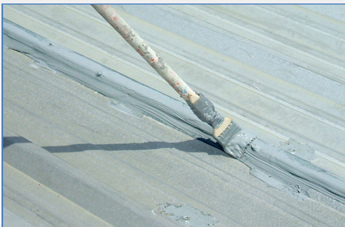
HER Polyurethane Sealant is applied to the seams, fasteners and penetrations and then smoothed with a brush.
